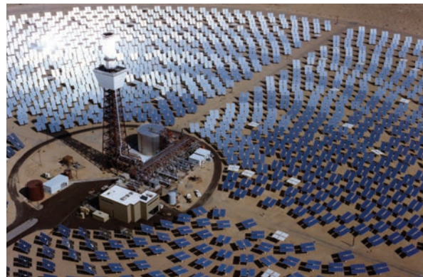
This solar power plant uses energy from the sun's light instead of from the combustion of fuel.
